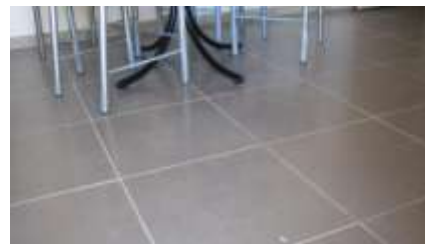
New tiles on the floor in cabin 4
