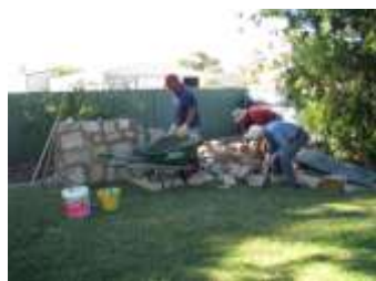
Building the Wall
